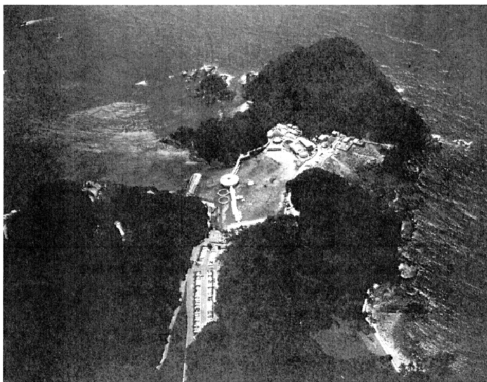
Fig. 1. Aerial view of Shimoda Floating Aquarium
